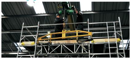
Aluminium beams which link two Access Towers to provide a large uninterrupted safe working area.
