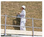
For use with our Super Board staging, these double guard rail and toeboard kits in lengths of 2.4m simply clamp on for ease of use.
