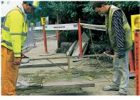
For small paving jobs and essential maintenance work you need this manual two man operational grab. It is ideal for removing small amounts of paving stones where you need a quick and safe solution.
