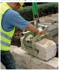
Scissor action grabs suitable for gripping kerb stones and L-shaped stones.
