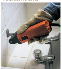
Remove discoloured grouting and damaged tiles with minimum effort. The oscillating blade reduces dust and guarantees precise cuts.
