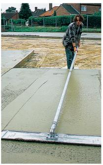
A float on a handle, this clever hand tool makes it easy to finish hard-to-reach areas of concrete such as those on large slabs and drives.
