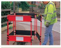
An all-in-one safety barrier, ideal for fencing off manholes, small excavations and similar hazards.
