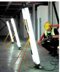
These 1.2m fluorescent lights with twin 36W bulbs can be linked together for illuminating large working areas or used individually for local, intensive lighting.
