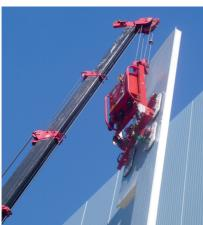
Dual circuit vacuum cladding lifters, specially developed for the safe, quick handling and installation of composite wall and roof panels. Multi-positional pads and a range of suction frames add
