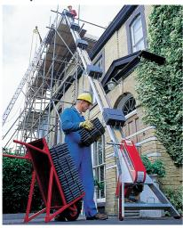
Safer and more efficient when you're bumping out a roof, this ingenious tile lift has been specially designed to get slates, tiles and blocks up to where they're needed quickly and with minimum effort.
