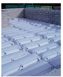
This Arrestor Bed is a Fall Arrest System which can be self-installed in most floor plans. The system will provide a practical adaptable solution particularly where the demands for fall protection are constantly changing.
