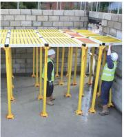
This compact, durable deck system is one of the UK's market leading fall prevention products. This compact, durable deck is designed to dramatically reduce your risks whilst working at height.
