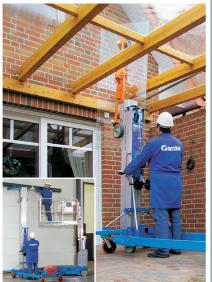
This counterbalance version of the Genie Super Lift Advantage allows you to raise loads up to 4.6m allowing you to work right up to walls. When fitted with the suction grip, large glass panels and windows up to 300kg can be installed into buildings without obtrusive base forks interfering in the installation.
