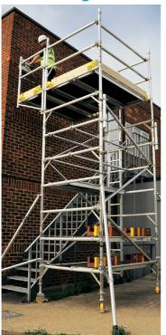
Conversion of a double-width Access Tower to provide access up to 1.25m outside the tower to overcome obstacles such as machinery, porches and stairways.
