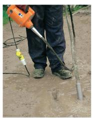
Portable, lightweight power units for fast compaction of wet concrete.
