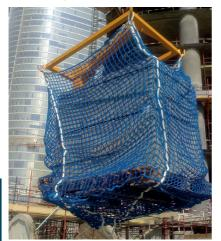
For handling palletised loads, this item saves you effort by allowing you to use an ordinary crane, in effect an ultra-high fork lift truck.
